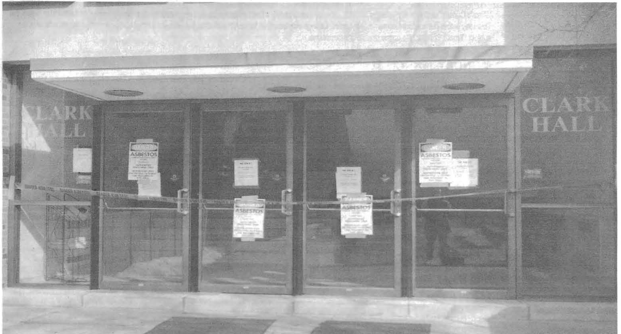
One of Clark Hall's entrances, marked with caution tape and warning flyers during the asbestos removal.
